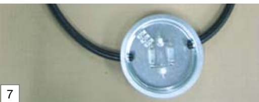
8. Empty pipe (steel ø 16 mm) as a cable duct longitudinally beneath the inner layer (from FP 38) 9. Lamp connection with pipe or with moulding to the inner area
