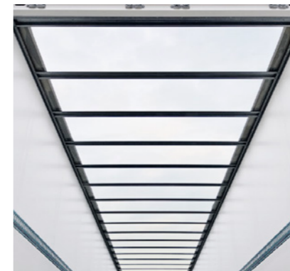
Light roof* for CEP services: translucent to allow day light to pass through.
