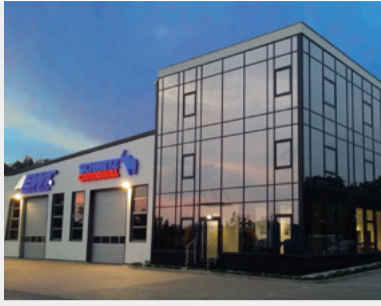
Trailer Center Gliwice, Poland
