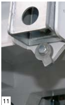
Corner stanchions from fine-grain galvanised steel, bolted, adjustable using eccentric cam
